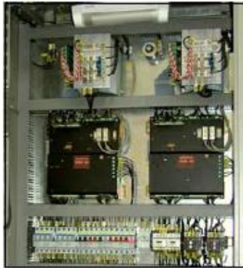
PRISMIC® A50 excitation system with a dual redundant control for a 90MVA turbogenerator
