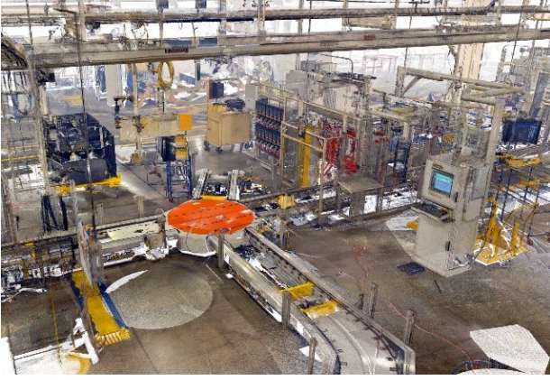
FIGURE 1. High-resolution industrial point cloud.
