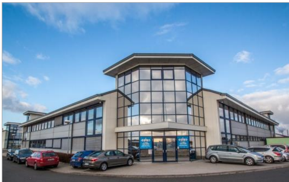
Fig. 1.3 One of the Safran Cabin CZ s.r.o. buildings in Pilsen [2]
