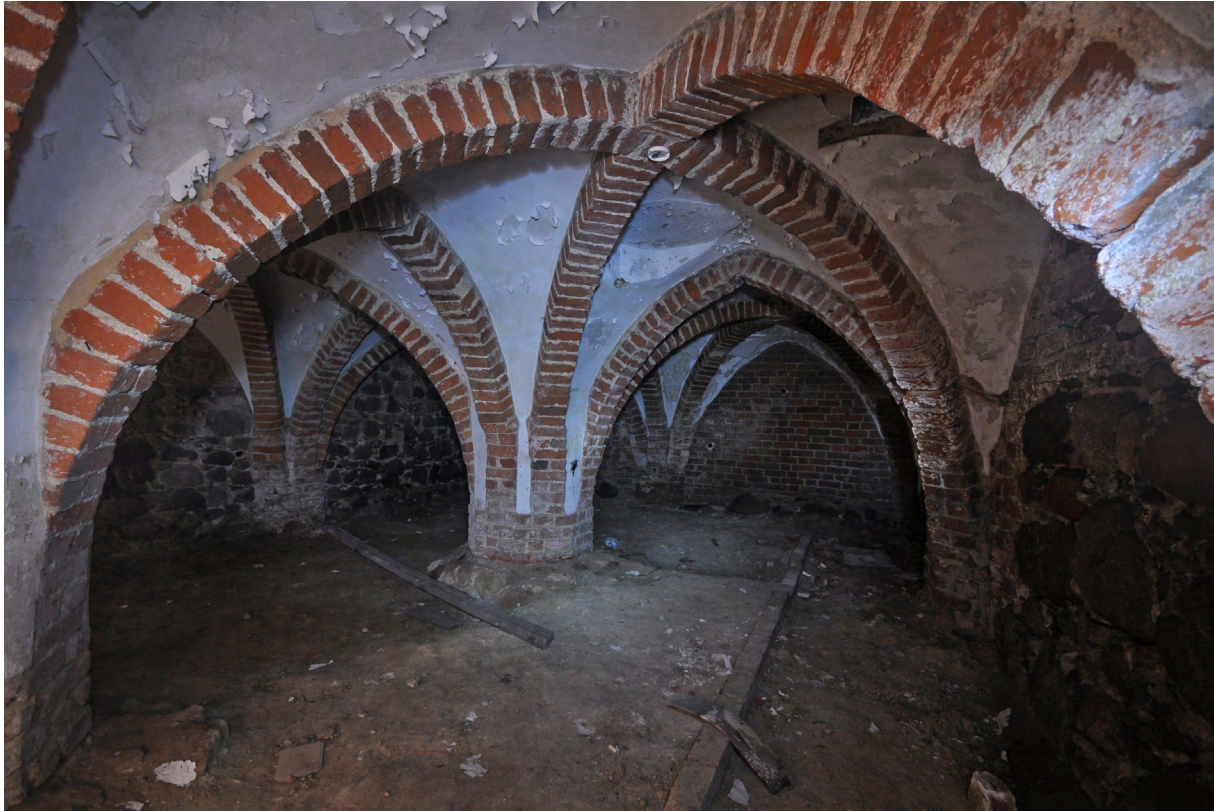
Fig. 13. Cellar of the south-western wing (photo B. Wasik).
