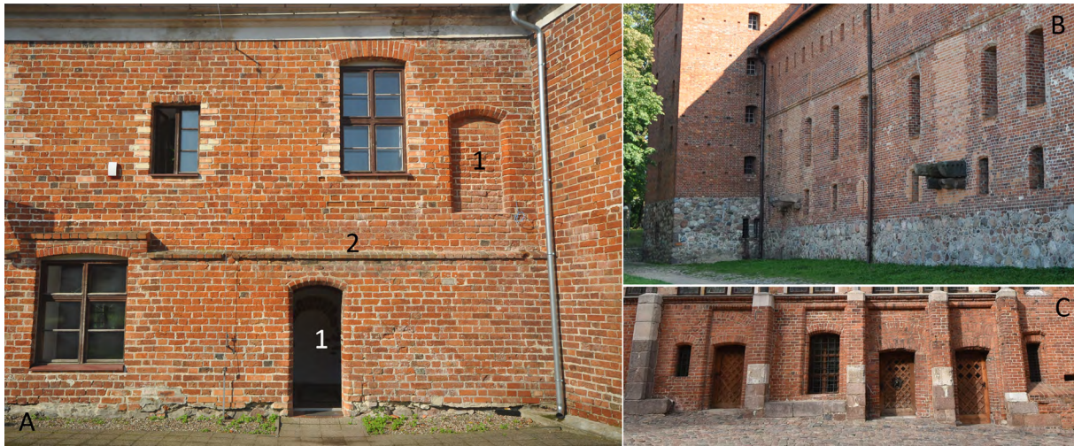
Fig. 8. Fragment of the south-western wing façade (A) with original entrance openings (1) and the offset on the gallery (2). The façade of the castle in Bytów (B) and the ground floor of the Grand Master's Palace in Malbork (C) (photo B. Wasik).
